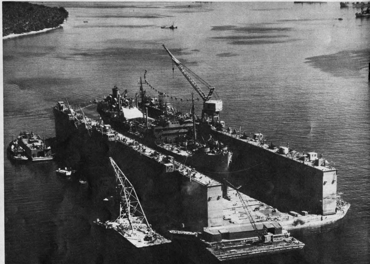
Bases away from home for our fleet are now outfitted with Navy's new floating dry docks. Shepherded by tugs, these mammoth structures are towed across the seas and are in operation almost before the
